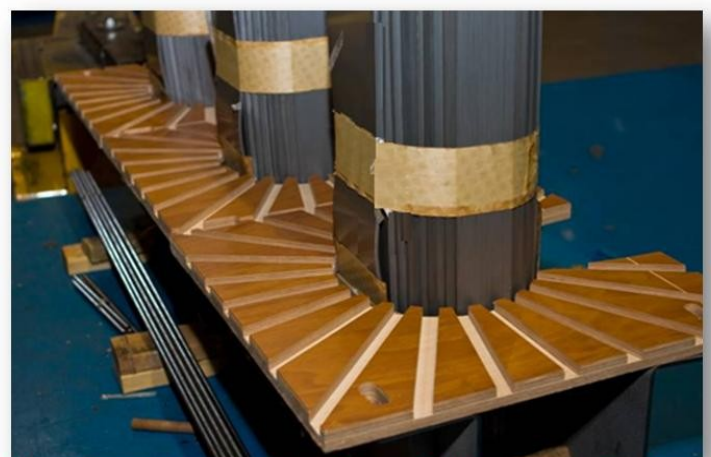
Lower Routed Pressure Plates Prior to Coil Placement on Core Legs
