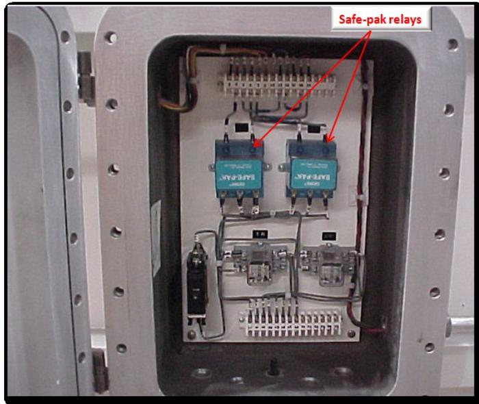
Adjacent is a close up photo of the previous image detailing the control enclosure. The enclosure serves as a centralized point in which to terminate the output from a variety of gauges and devices located on the transformer including liquid level gauge, thermometer, pressure vacuum gauge, and sudden rise pressure relay. The outputs from these devices control the operation of connected equipment, largely through relays. To prevent the
