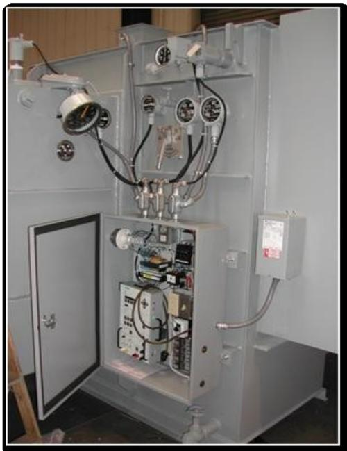
site. Note that the wiring from the various gauges is exposed SO cable. Entrances to the terminal box are made via watertight connections. The terminal box enclosure itself provides a degree of protection against:
