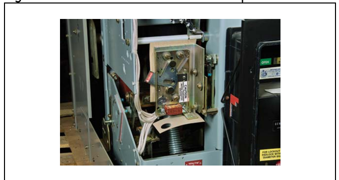
Figure 8: AKR Circuit Breaker without Trip Unit
