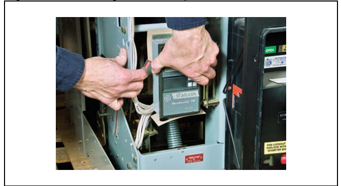
Figure 7: Removing the Old Trip Unit
