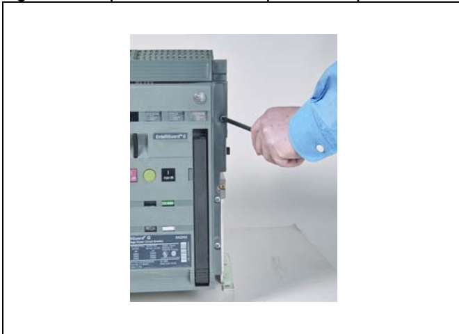
Figure 10. Trip Unit Removal Sequence, Step A
